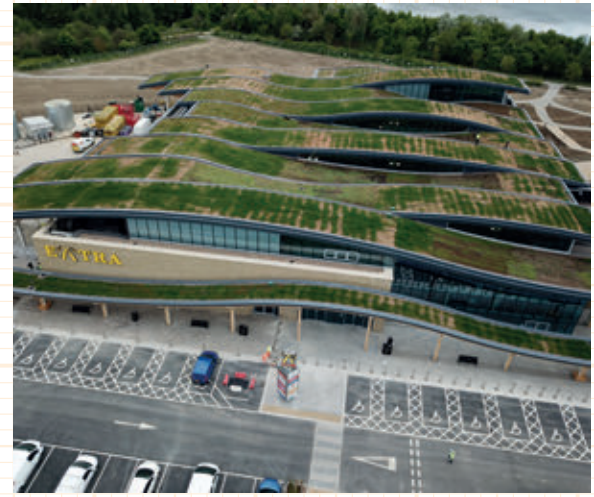
Figure 11: Aerial photo of Leeds Skelton Lake services 150
