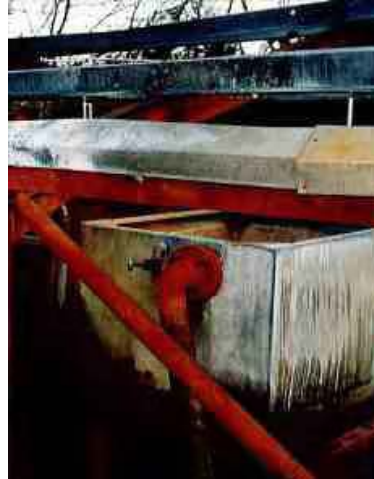
Figure B.28 Minimally damaged lightweight tanks and housings in the pump house where the explosion started.
