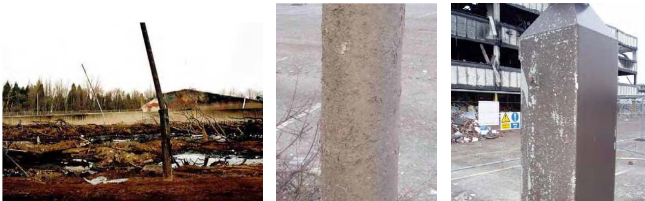
Figure B.31 Effect of drag forces on a lamppost (left), and abrasions to objects in the car park: the base of a tree (middle) and on a steel post on its south face (right).
