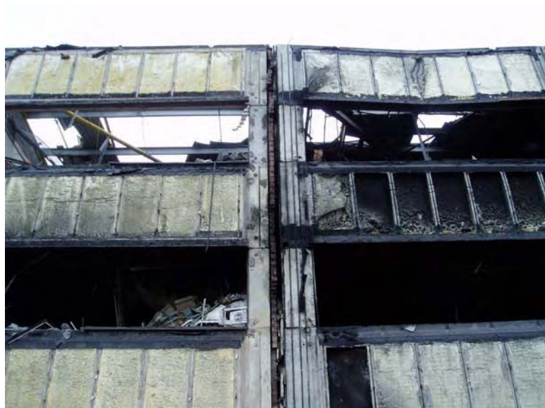
Figure 8 “strong” (left hand side) and “weak” (right hand side) cladding panels on East face of the Northgate Building
