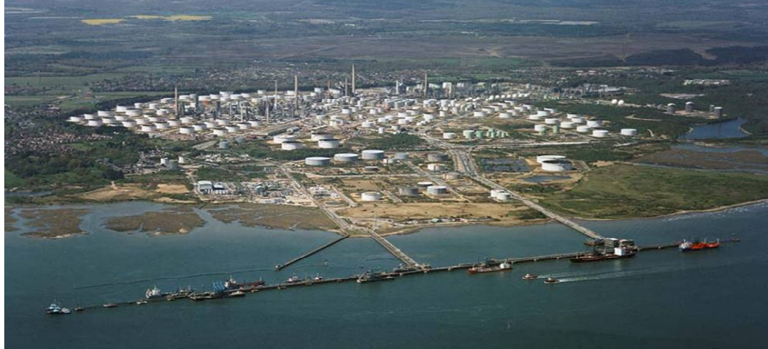
FIGURE III-2 FAWLEY REFINERY—SHOWING PROCESS UNITS, TANK FARMS AND JETTY
