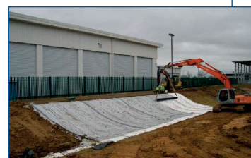
Containment improvement using bund liners
